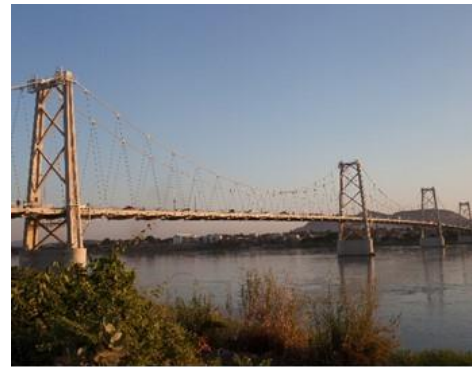
Fig.1: The longest suspension bridge in Africa linking Maputo with the Catembe district
