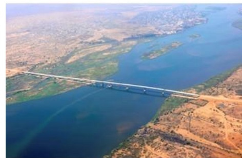
Fig.2: The second bridge over the Zambezi River in Tete
